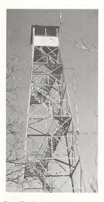
Figure 250. Signal Peak lookout, an Aermotor MC-39, on the Tonto National Forest.
